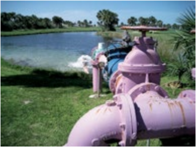
Reclaimed water pipes are painted purple for easy identification.
