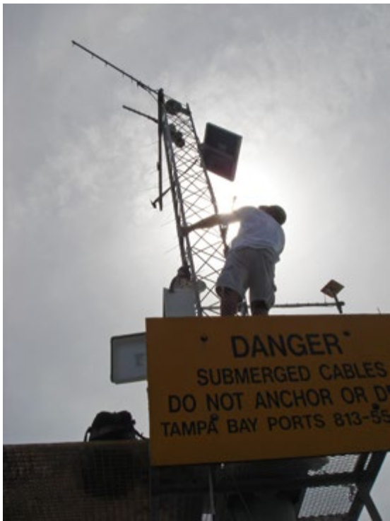
A PORTS tide monitoring station at Port Manatee. The PORTS network collects real-time information on winds, tides and currents to improve safe navigation for mariners. Photo by Mark Luther.
