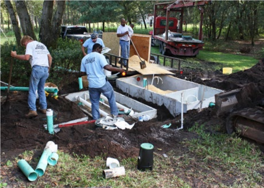
A “passive nitrogen reduction” septic system utilizing bio-filters was installed and field-tested in 2015 at a residential site in Hillsborough County. Photo courtesy Florida Department of Health.
