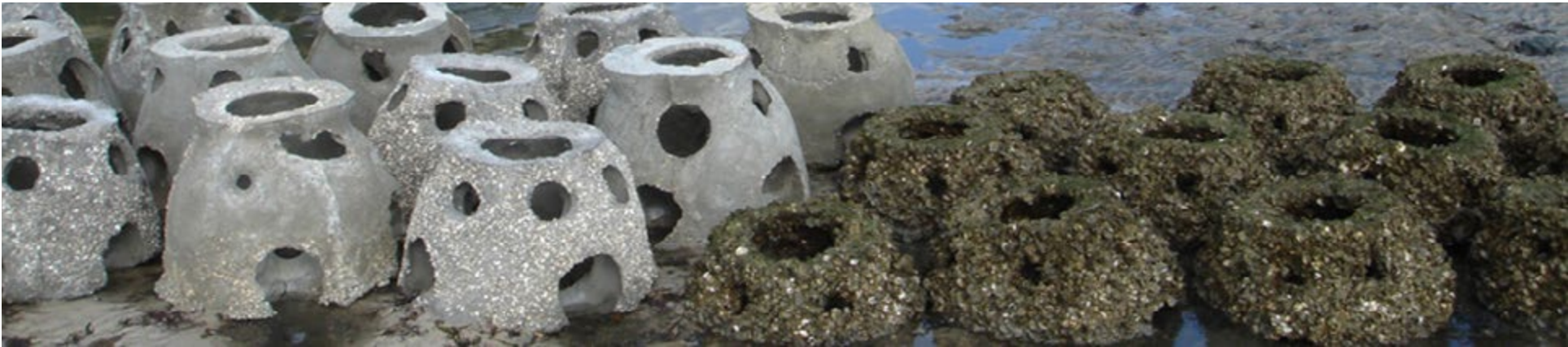
Concrete oyster domes placed in front of seawalls provide a substrate for oysters, barnacles and other encrusting organisms to attach. Photo courtesy Tampa Bay Watch.
